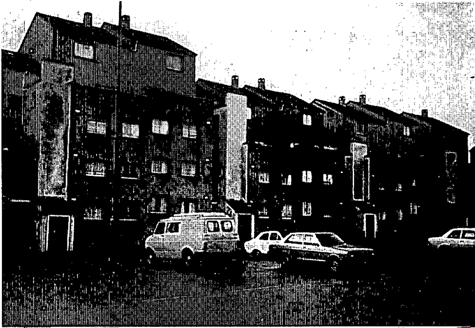
FIG 1.5 House 7 : first floor flat ('X' shows the location of mould growth; see section 3)
