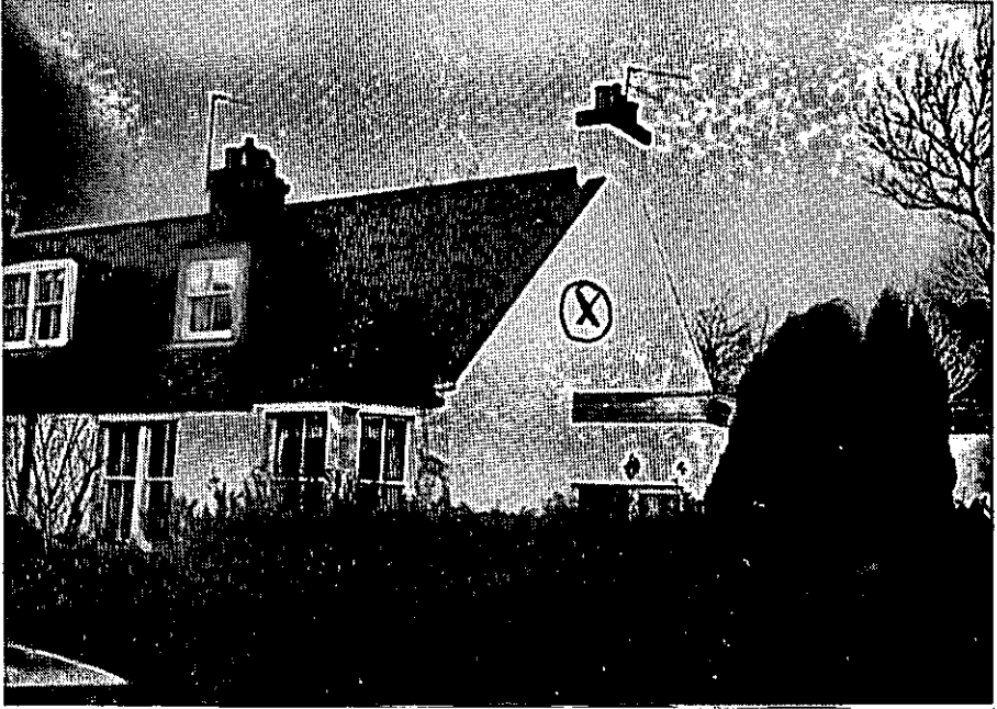
FIG 1.1 House 1 : end terrace 19th century ('X' shows the location of mould growth; see section 3)
