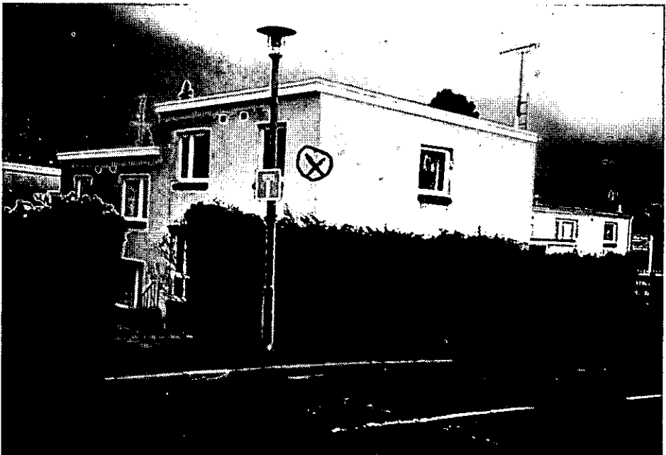
FIG 1.4 House 6 : end terrace/detached house ('X' shows the location of mould growth ; see section 3)
