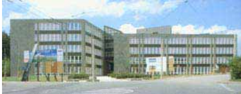
Figure 11: Overall view of the Sarinaport building from the south-east
