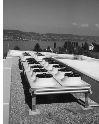
Figure 13: Air coolers on the roof contaminated to the workplace. By this means very good ventilation efficiency is achieved.
