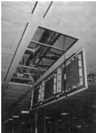
Figure 8: Installation of chilled ceiling panels
