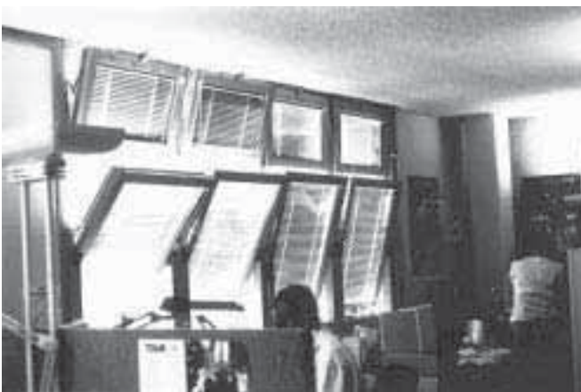
Figure 3: Internal views of office layout showing centre pivot windows below, bottom-hung hopper windows in the upper part
