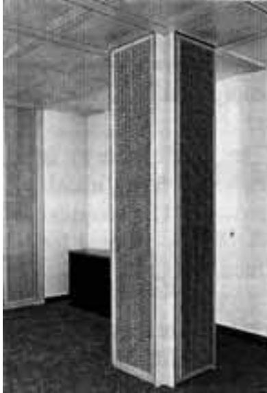
Figure 6: View of displacement ventilation outlet. Air flow 100 \text{ m}^3/\text{h} per side, total 400 \text{ m}^3/\text{h}
