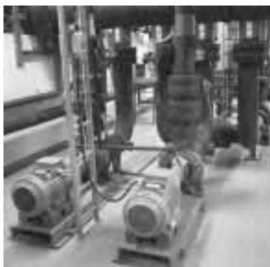
Figure 6: The ground water pumps in the plant room
