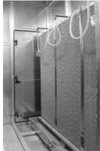
Figure 12: Evaporative humidifier
