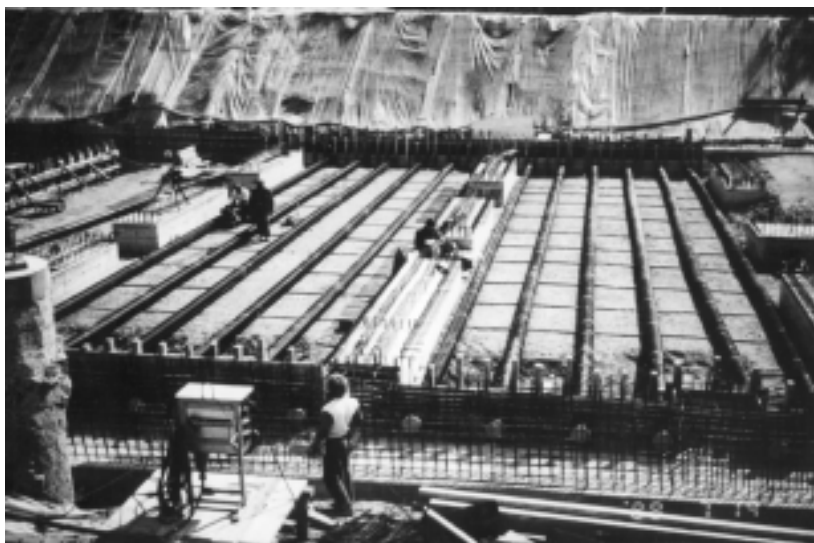
Figure 9: View of the ground coupled system during construction. At the front and rear of the picture, the accessible concrete ducts are seen under construction. At the right, the plastic pipes may be seen after covering with gravel.
