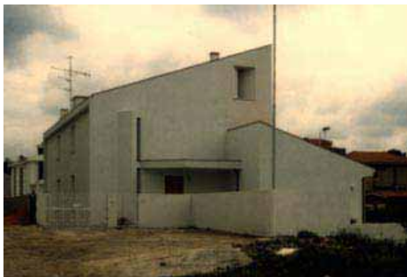
Figure 13: View of the North and West façades of the residence
