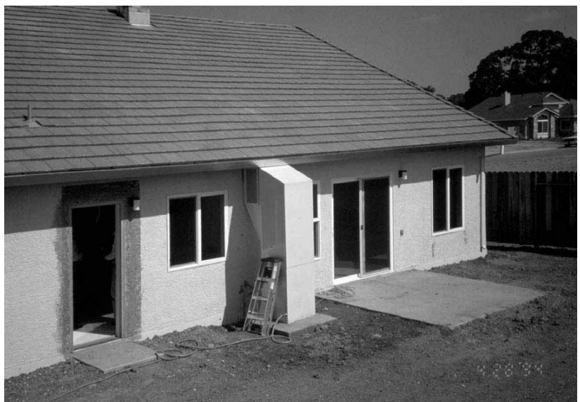
Figure 6: South elevation showing evaporative cooler
