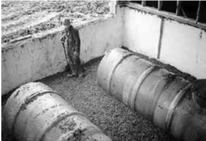
Figure 8: Installation of the rainwater storage tanks under the garage slab
