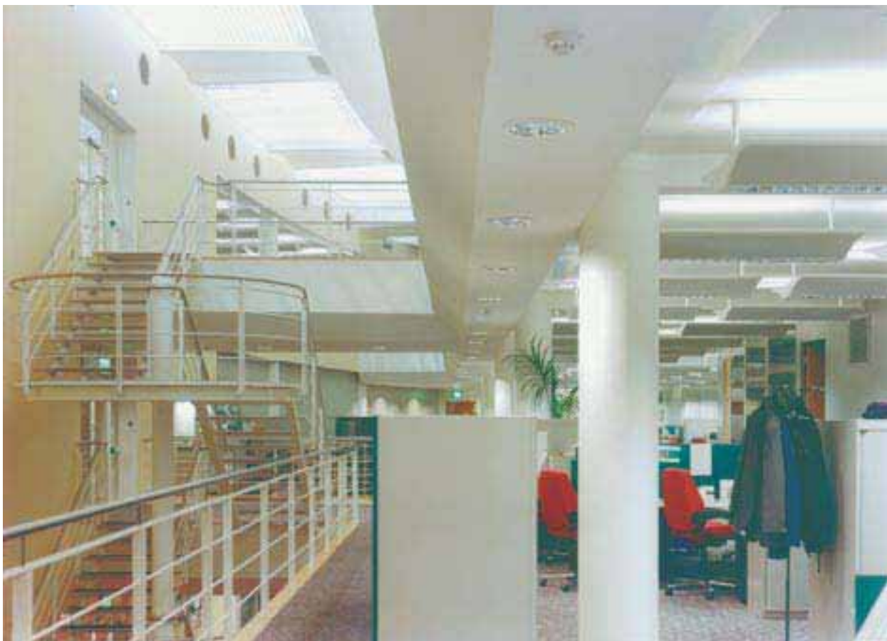
Figure 7: Natural light penetrates the space and uplighters are photo-electrically controlled
