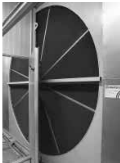
Figure 5: The rotary desiccant wheel
