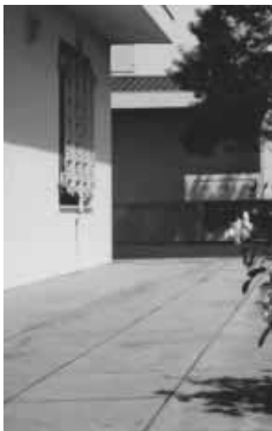
Figure 8: Structural overhang for shading the south-facing windows
