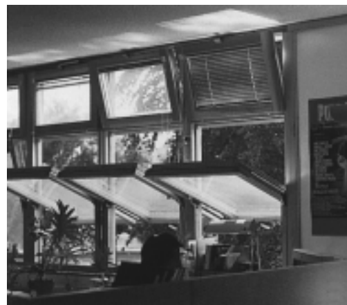
Figure 3: Internal views of office layout showing centre pivot windows below, bottom-hung hopper windows in the upper part
