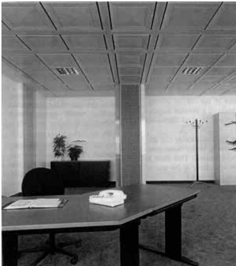
Figure 5: View of retrofitted office with chilled cassette ceiling and displacement ventilation system
