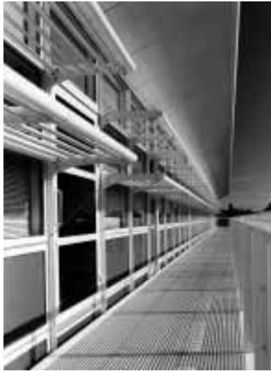
Figure 3: Solar shading on the southern façade
