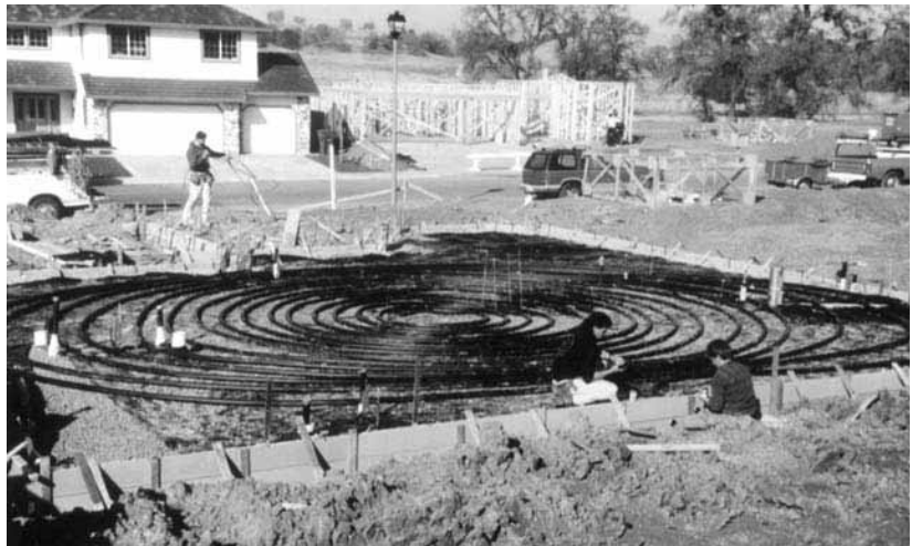
Figure 6: Plastic tubing being installed
