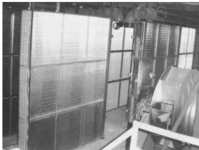
Figure 2: One of four plug fans and coil bank during installation
