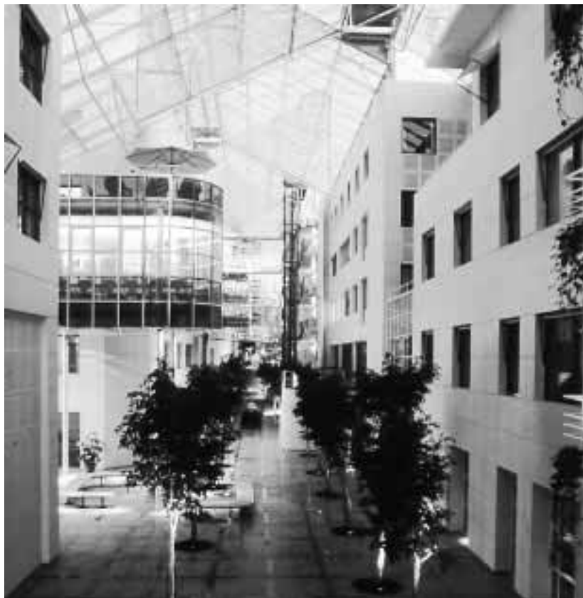
Figure 2: The "Interior Street" is ventilated by overflow air from the offices
