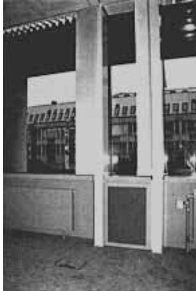
Figure 7: View of radiator and façade displacement ventilation outlet. Air flow 100 \text{ m}^3/\text{h}
