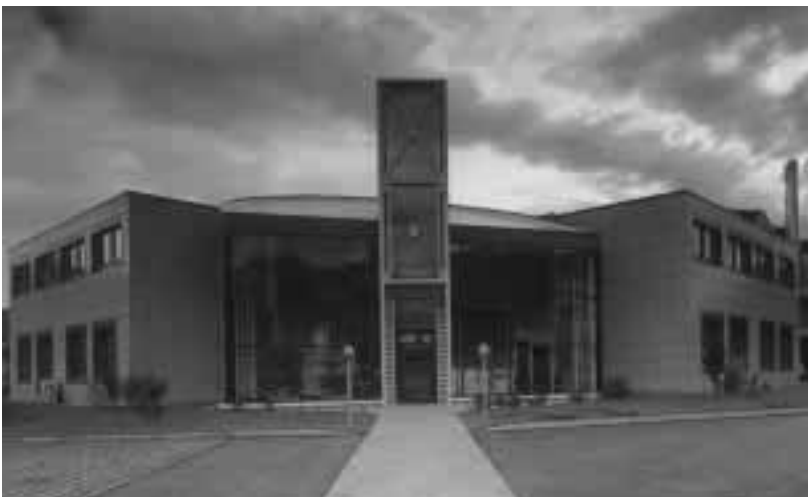
Figure 1: The Schäublin SA administration building in Delémont was the first building to be based on the BATISO ® principle
