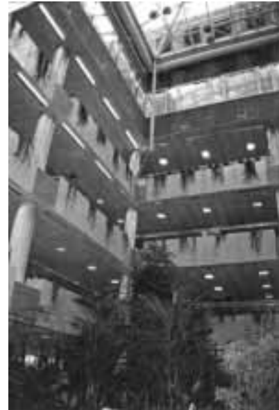
Figure 4: Atrium with open access to the office floors
