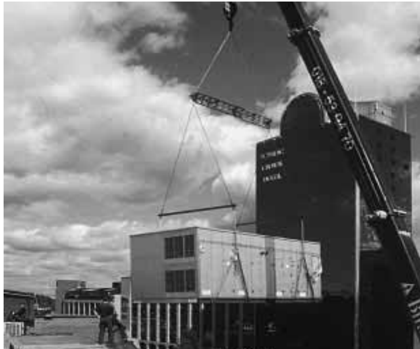
Figure 4: The unit was lifted on to the roof ready for operation
