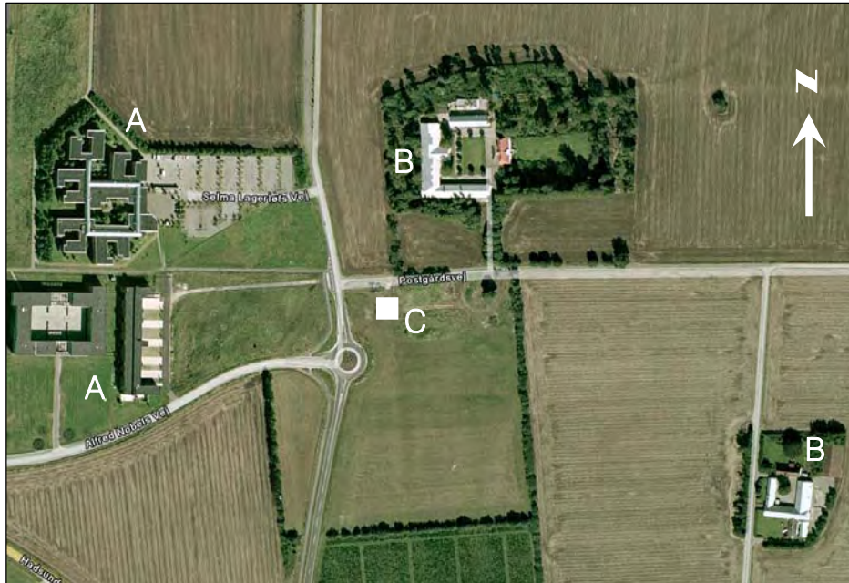
Figure 1. Site location of 'the Cube'. A – three storeys company building, B – one storey farm, C- 'the Cube'.
