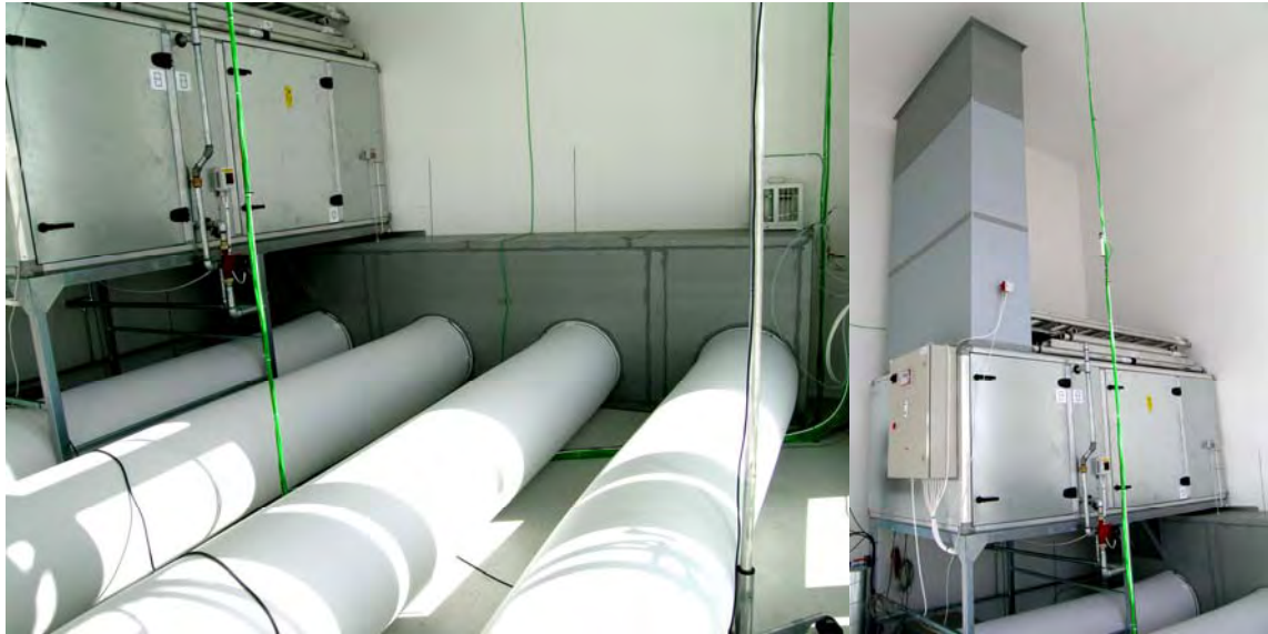
Figure 17. Ventilation recirculation system.
