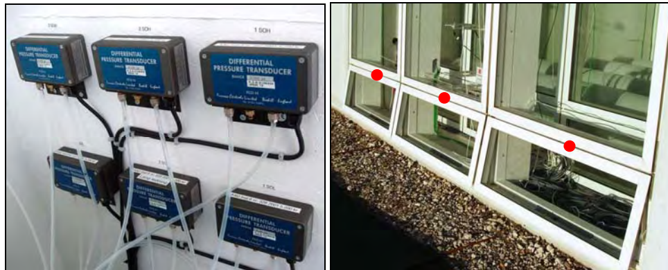
Figure 39. Pressure transducers Furness Controls Ltd. FC044 (left). Location of the pressure measurements at the window surfaces, SOL-openings (right).
