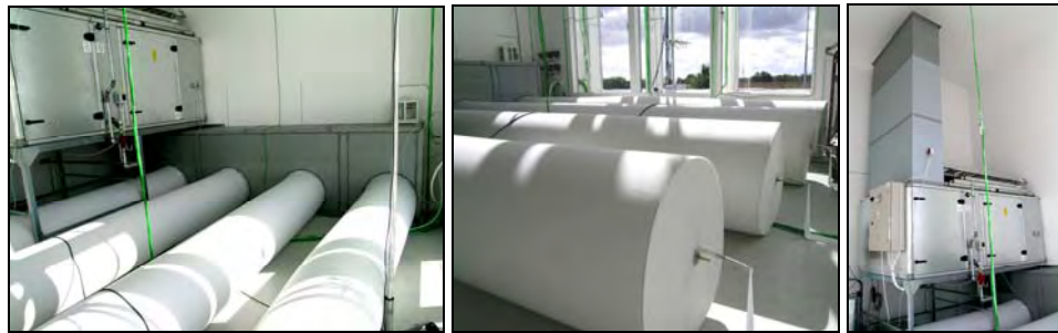
Figure 4. Ke-low impulse ducts (left, centre). Ventilation system in the experiment room (right).
