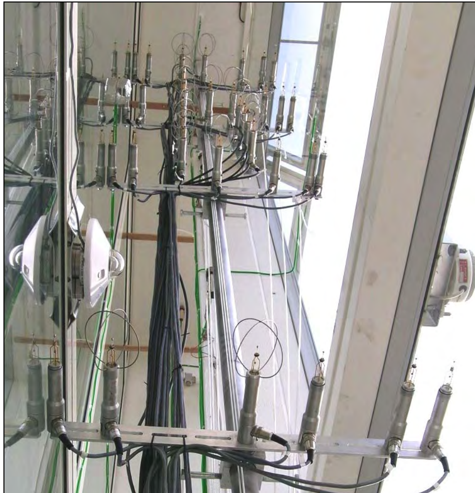
Figure 36. View to the final positioning of anemometers in the cavity (view from the bottom of DSF).
