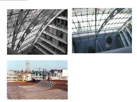
Figure 5.44 - Berliner Bogen: example of the building construction — double skin facade and floor slabs, winter garden and installation of the pipe-work [www.uponor.de/(August 2008)].
