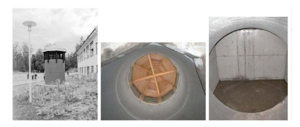
Figure 6.18 - Jaer School air intake tower (Left: outside, Middle: inside looking up, Right: inside horizontally into base of the tower from the horizontal ETAHE duct.) [Schild (2002)].
