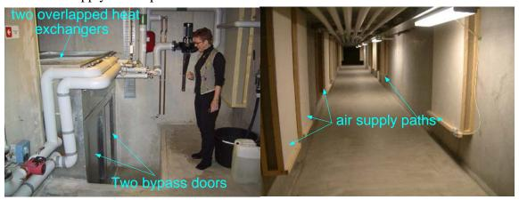
Figure 6.15 - Air distribution duct of Mediå school (Left photo shows heat exchangers and "summer" doors. Right photo shows the supply air paths) [Tjelflaat (2002a)].
