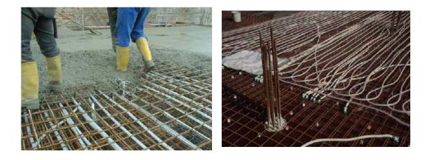
Figure 5.9 - Concrete lying on the reinforcement grid with attached pipes [Hauser et al. (2005)].
