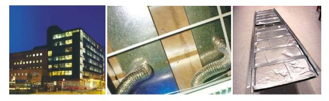
Figure 7.20 – Picture of the "Stevenage Borough Council" building – Construction details of the PCM based ceiling (Cooldeck technology).
