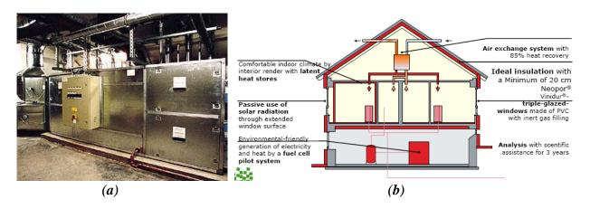
Figure 7.16 - "3-Litre" house - (a) Air handling unit and heat recovery - (b) main features of the energy retrofit.
