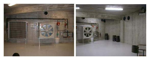
Figure 6.19 - The air distribution room, showing the preheat unit (left) and fan, as well as the plastic subterranean ducts leading to the various rooms [Schild (2002)].
