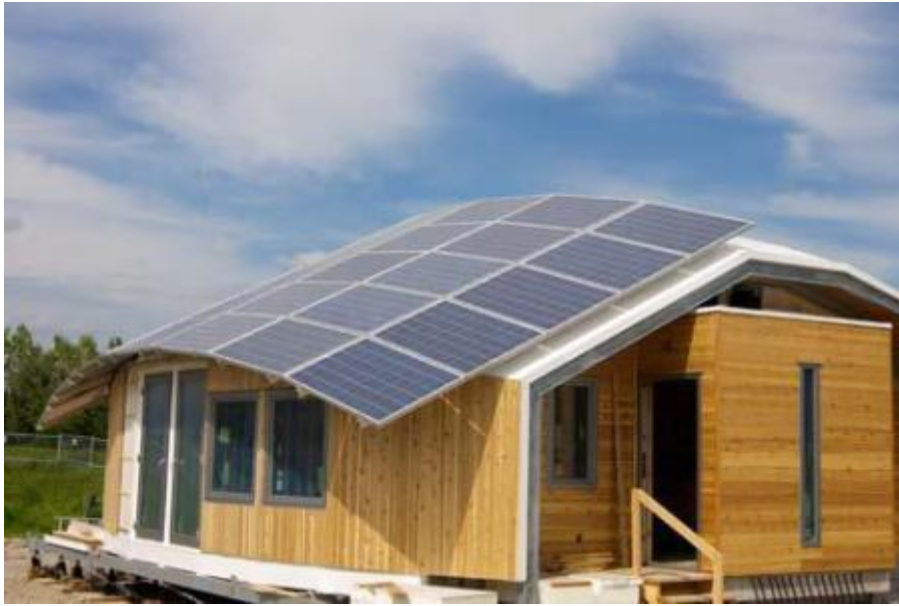
Figure 2-7: Building Integrated Photovoltaic System in Canada by Schletter and SkyFire with “turtle” roof shape [2-10]
