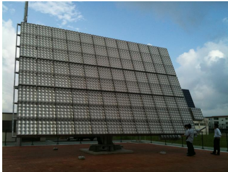
Figure 2-8: CPV with dome shaped lenses
