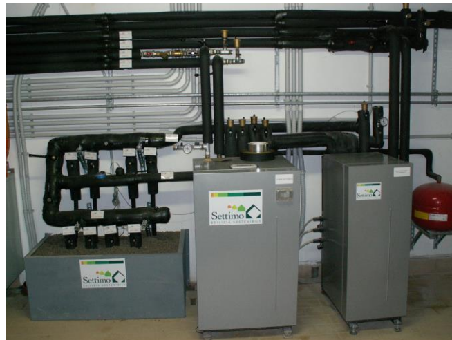
Figure 2-10: A GSHP, centre, left connections with two boreholes with two tubes each, right the free cooling unit
