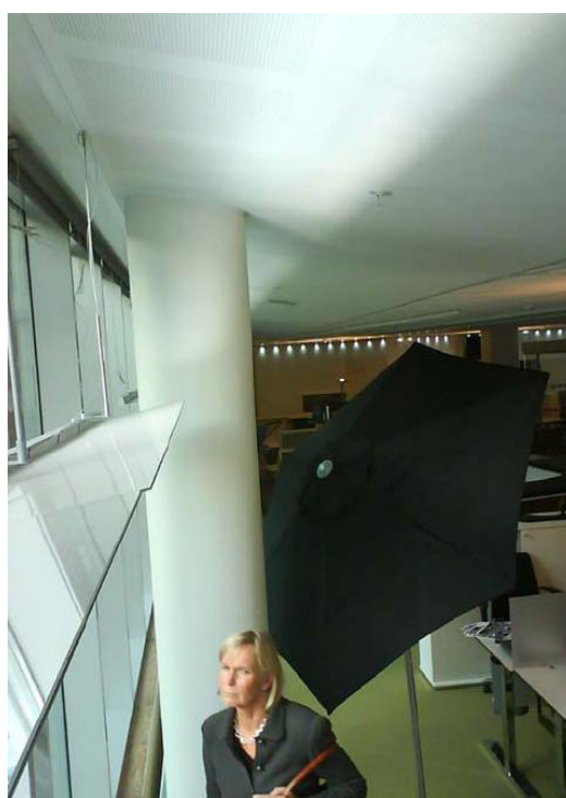
Light shelf with integrated LED light sources
